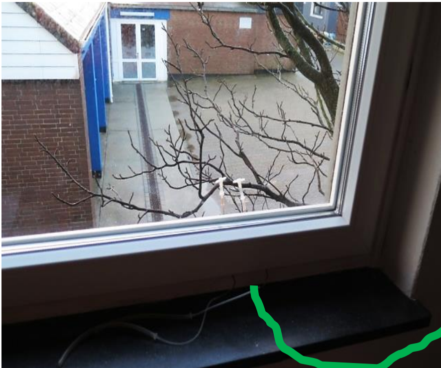
Measurement of the pressure difference on an exterior wall
